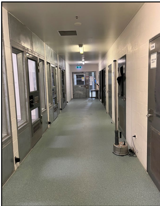
3. Reception corridor containing dry cell, reception holding cells and video link rooms (photo taken at night).
