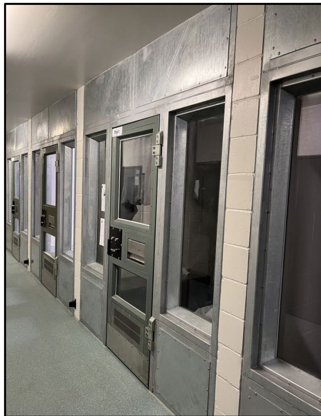
4. Reception corridor with dry cell on the right. Note the prisoner's jumper being used to partially cover up the door's top window (photo taken at night).
