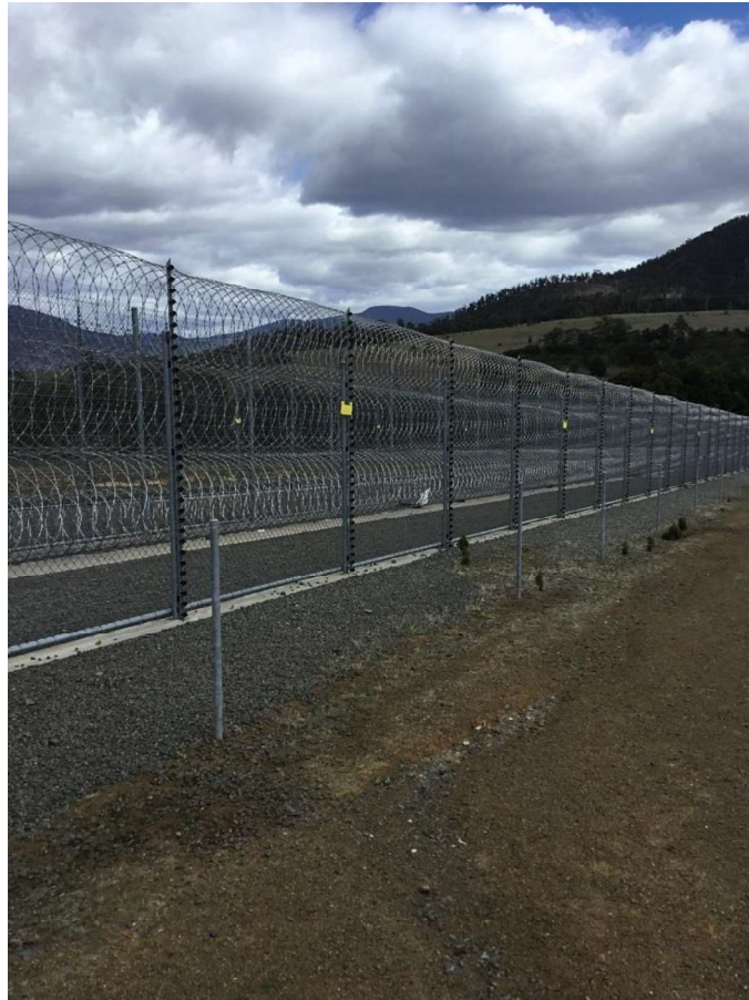
Risdon Prison Complex perimeter fence
