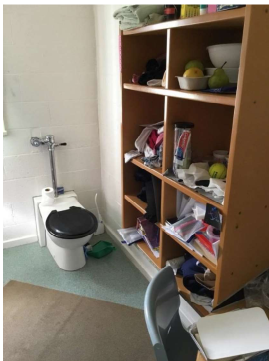
Mary Hutchinson Women's Prison bunked cell – no privacy screens
